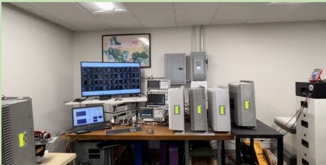
5 VSMs working with two PV simulators and one BYD battery
